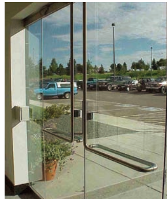
Retrofit installation of Smart Touch replacing mechanical panic
